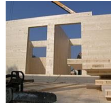
Wooden wall construction
