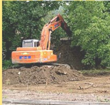
Extraction of clay plaster
