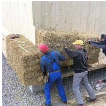
Straw bale wall construction
