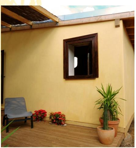
strawbales, clay and lime mortar with olive oil additive for water proofing (without compromising vapor difusion)
